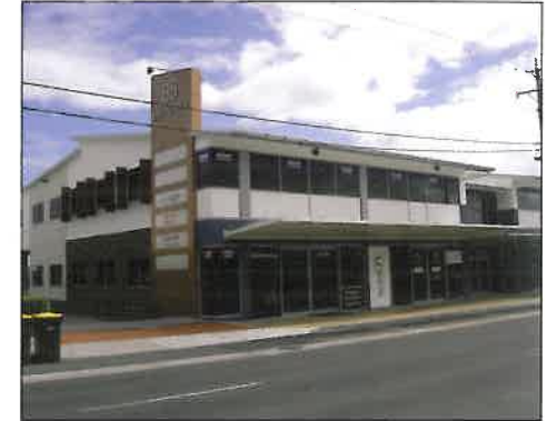
Commercial Buildings (Office Accommodation) up to $4 million Builder Rhind Constructions Pty Ltd Project Devenio Phone 4194 6270 www.rhind.com.au
